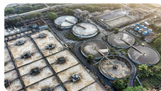
ZLD / MLD Wastewater Treatment
